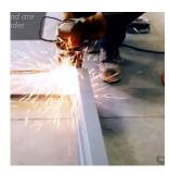
If you are installing a welded frame, remove the shipping spreader bar 5. before placing the frame in the opening. Note: Temporary shipping bars must be removed and are NOT to be used as spreader bars to set the frame.
