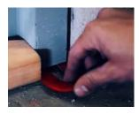
8. Verify that the head is level. If it is not level, shim under the bottom of the frame.
