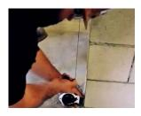
6. Make a mark at the top and the bottom of the masonry wall. Snap a chalk line between the two marks. Set the frame into the opening using the chalk line on the wall to locate it.
