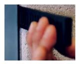
9. Shim at the bottom of the frame, keeping the hinge side tight to the wall and adding shims to the lock side to tighten the frame to the spreader bar. If more than a ¼" shim is needed, divide the amount of shims evenly between the two jambs. Make sure all four rabbets of the frame touch the spreader bar. This will prevent a twist in the frame.
